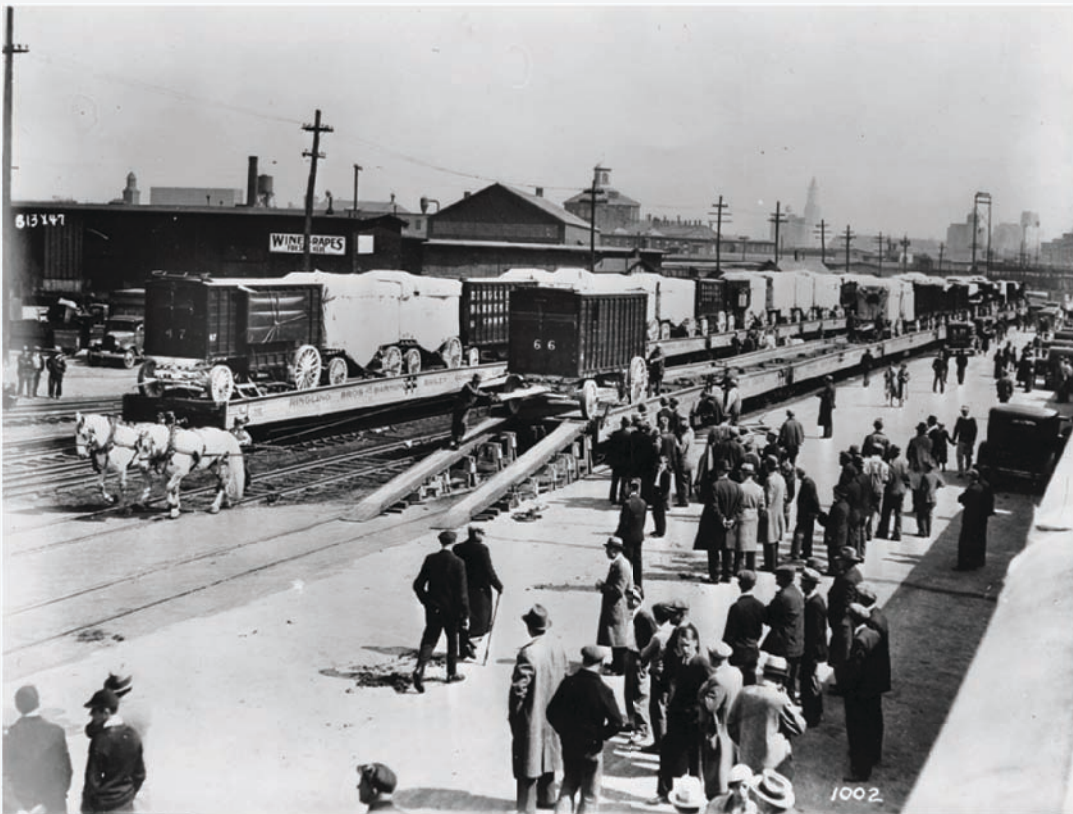
FIGURE 3: Flat Car Unloading
